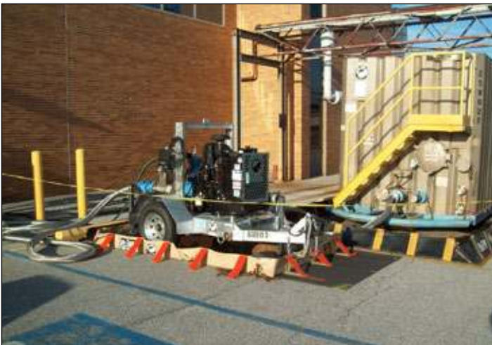
Some jobsites required stainless steel tanks and hose during the turnaround.
