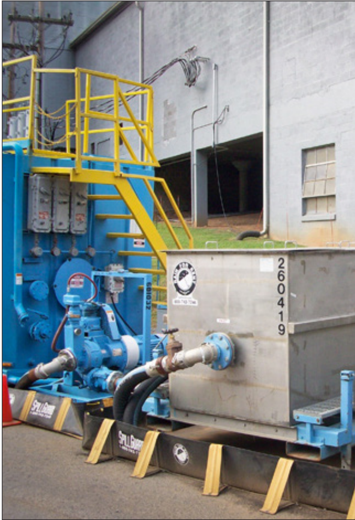
Temporary bypass performs beyond expectations over two years.
