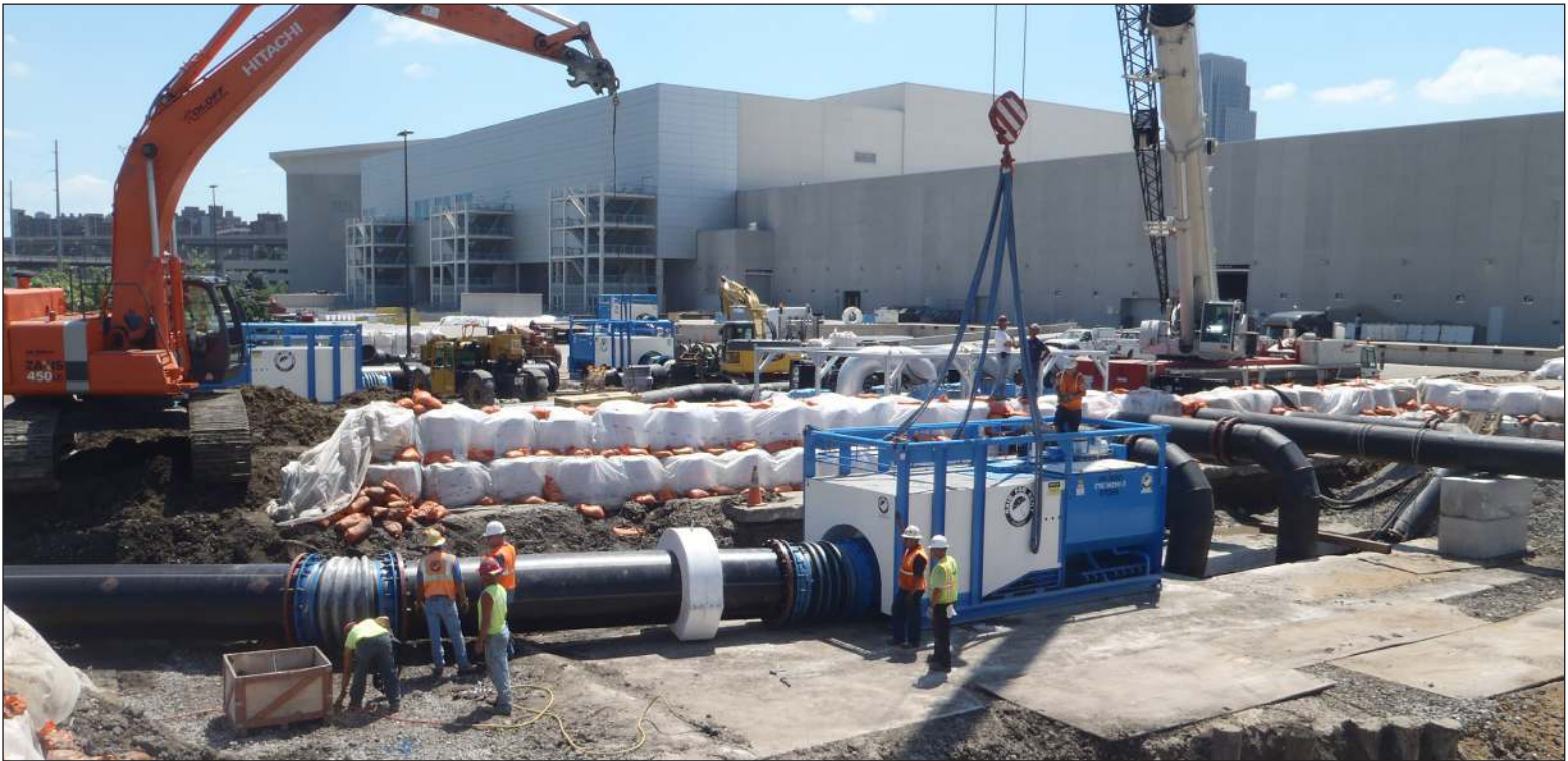
Rain for Rent crews install the first FP-1050 42" Axial Flow floating pump into the newly constructed temporary CSO suction pit.
