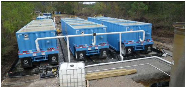
Polymer injection and media filtration treated polluted water on site.
