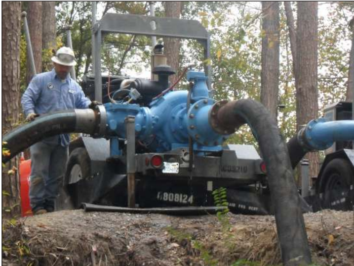
A 7000 GPM average creek bypass was designed to allow remediation along a 2400 foot section of contaminated creekbed.
