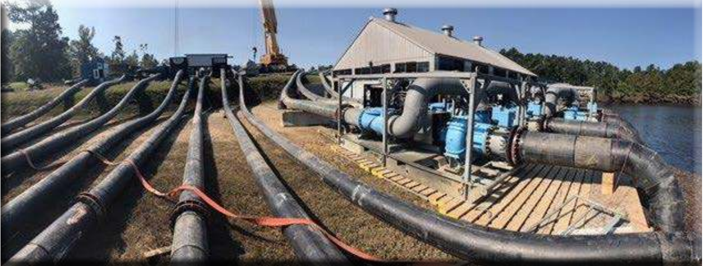
Rain for Rent DV600c bypass system - Beaumont TX - Hurricane Harvey Response
