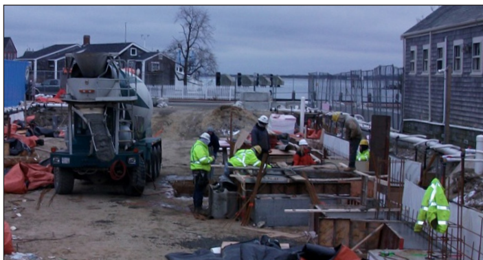
Dewatering was a crucial aspect to ensure a solid foundation.
