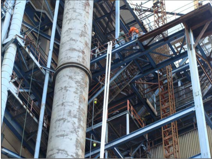
The hydrocleaning contractor was able to reduce the amount of offsite waste transport thanks to the filtration system from Rain for Rent.
