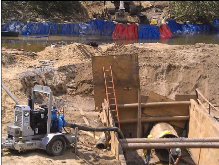
Dewatering provided stability needed to continue directional drilling.
