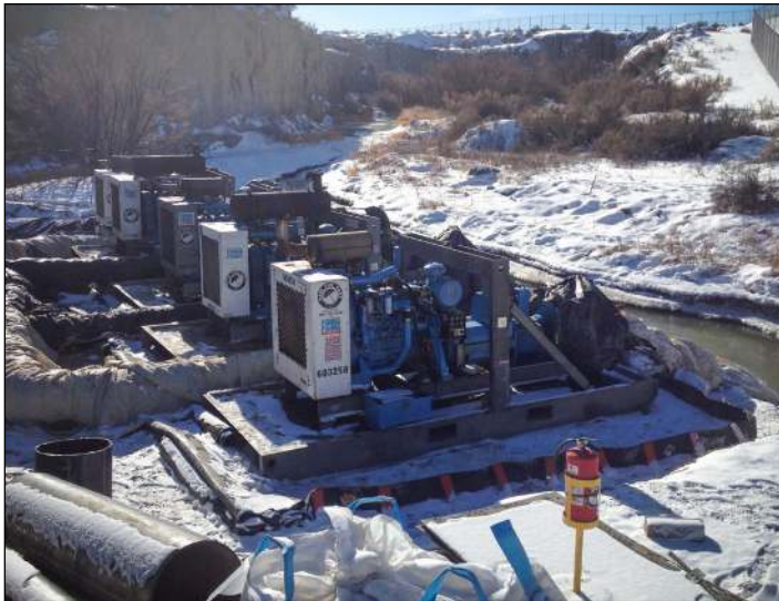
Five DV300i pumps moved 22,000 GPM in sub zero temperatures.
