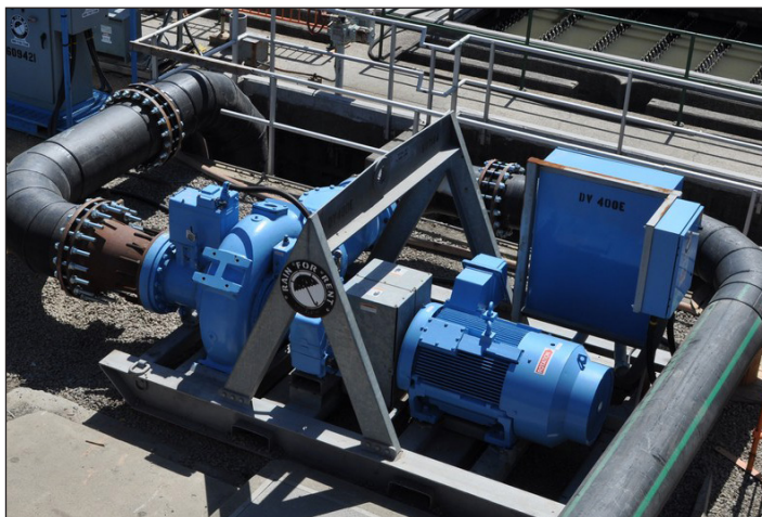
Four DV400 pumps were used to bypass flows up to 56 MGD .
