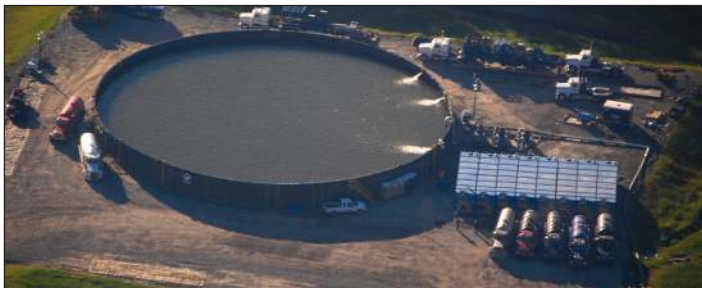
This frac site pumped water from the LakeTank at 100 BBL per minute.
