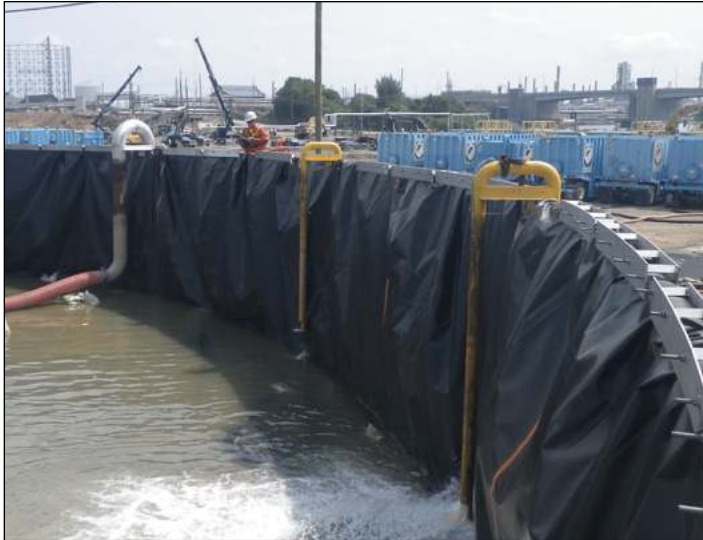
Dewatered water was pumped into the LakeTank to hold for filtration.
