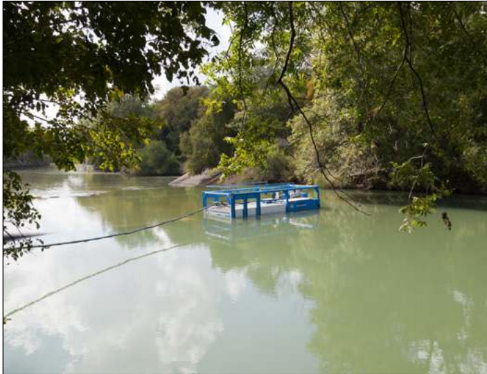
The FP1050 axial flow pump was floated in the river to provide the 90 MGD bypass flow needed to keep residents supplied with water.
