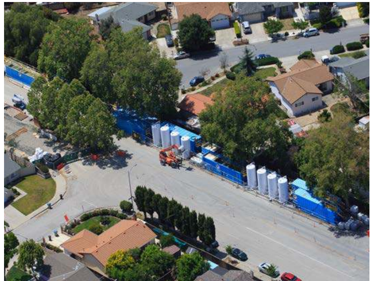
10K# carbon vessels filter for 160,000 ppB VOC C5 thru C12, Sierra at Lunde.
