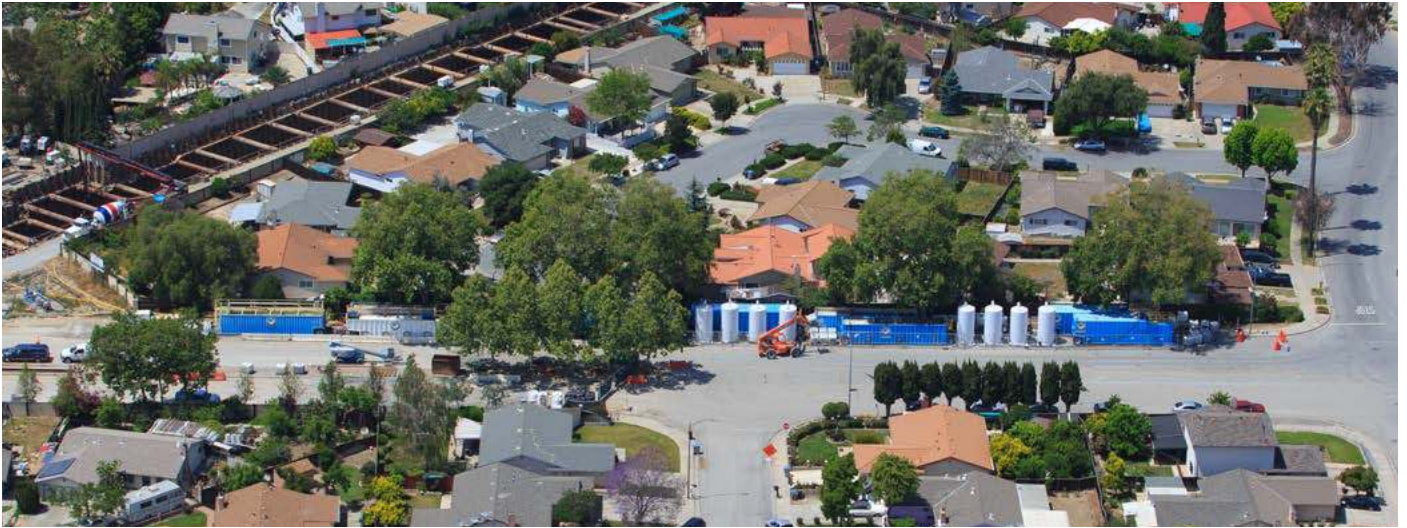
10K# carbon vessels filter for 160,000 ppB VOC C5 thru C12, Sierra at Lunde.
