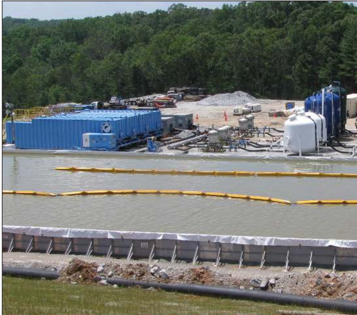
The 800,000 gallon MOD tank in the foreground allowed for settling of contaminants pumped from the SMU. The effluent then went on to additional polishing. The frac tanks supplied clean water for backwash.
