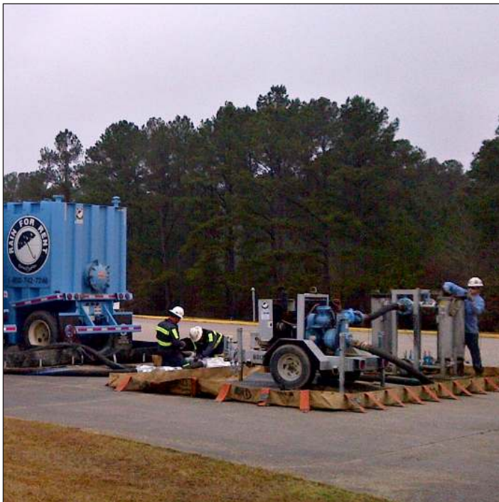
A pump and filtration system was used to meet discharge requirement standards and reduce waste disposal costs for the pipeline service company.
