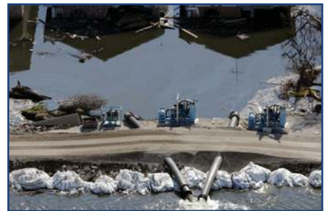
Temporary pumps moved floodwaters through the repaired 17th Street Canal Levee in the aftermath of Hurricane Katrina in New Orleans.
