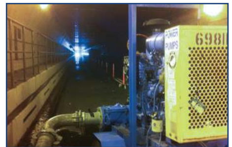
Temporary pumps moved floodwaters through the repaired 17th Street Canal Levee in the aftermath of Hurricane Katrina in New Orleans.
